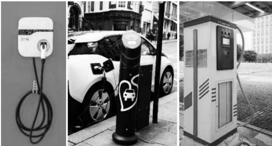
A domestic wall-mounted charging point, a floor-mounted charging point, and a rapid charging point
